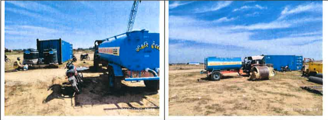
Drinking water facility provided at construction site
