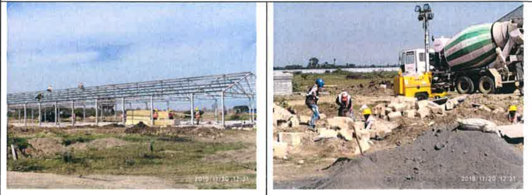
Construction workers using PPEs
