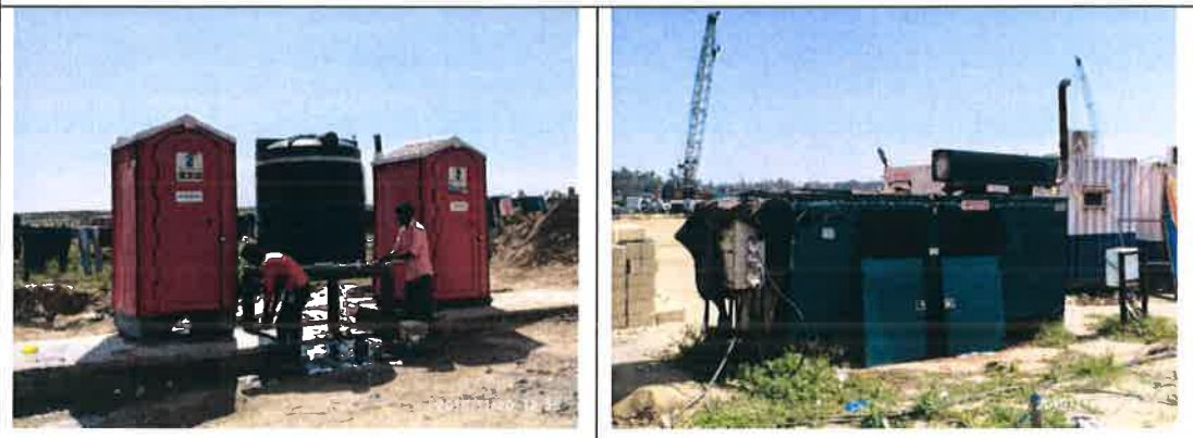
Sanitation facility at Construction site
