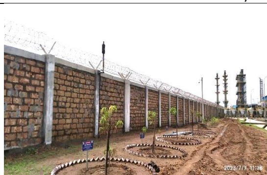
Boundary wall with CCTV surveillance and Intrusion detection system
